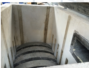
The unique hearth bar technology allows for efficient incineration from above and below.
